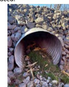
Culvert #10: 800 mm CSP. Proposed to be replaced.
