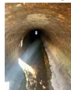
Culvert #7: Lined, 600 mm CSP. Proposed to be replaced.
