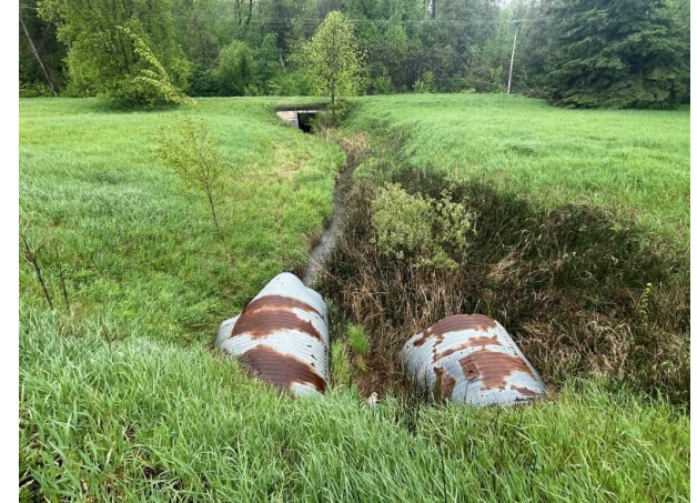
Culvert #9: Corroded, twin 1600 mm CSPs conveying the Morrow Branch of the Cumming Drain. Proposed to be replaced.
