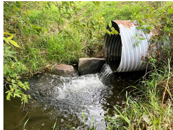
Culvert #11: Perched 900 mm CSP, east of the Maxville Manor. Not proposed for replacement. Recommend river run rock outlet.
