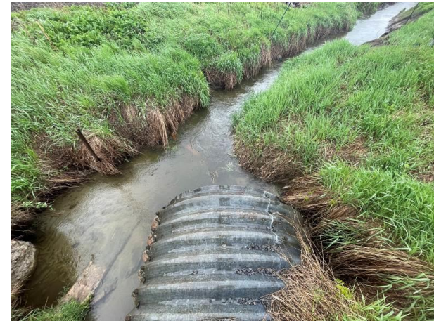
Culvert #6: Damaged, 1600 mm CSP with erosion issues conveying Cumming Drain. Proposed to be replaced.
