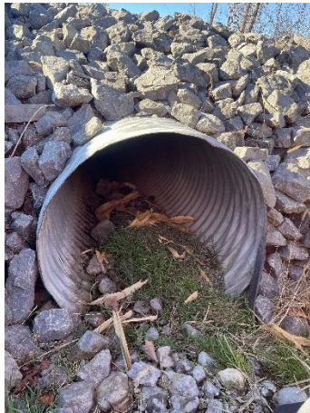
Culvert #10: 800 mm CSP. Proposed to be replaced.
