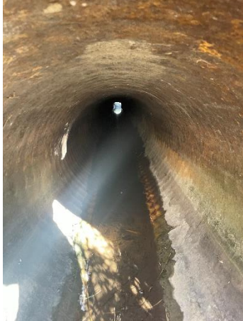
Culvert #7: Lined, 600 mm CSP. Proposed to be replaced.
