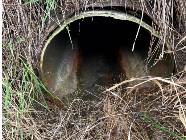
Culvert #8: Lined 600 mm CSP, 40 m west of Cumming Road. Proposed to be replaced.
