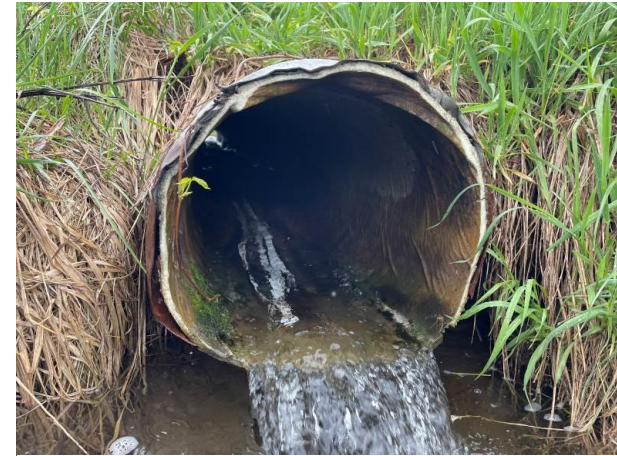
Culvert #3: Lined and perched 500 mm CSP, west of Fraser Road. Proposed to be replaced.
