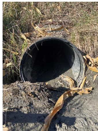
Culvert #5: 600 mm HDPE pipe. Not proposed for replacement.
