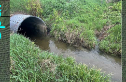
Culvert 8: 500 mm Ø CSP plus liner
