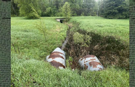
Culvert 9: Twin 1600 mm Ø CSP
