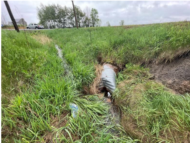
Culvert #1: Damaged, 600 mm CSP immediately east of Highway 138. Proposed to be replaced.
