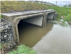
Culvert 4: Twin box culverts 38 m Steel Beam 3.3 m wide x 2.4 m ht.
