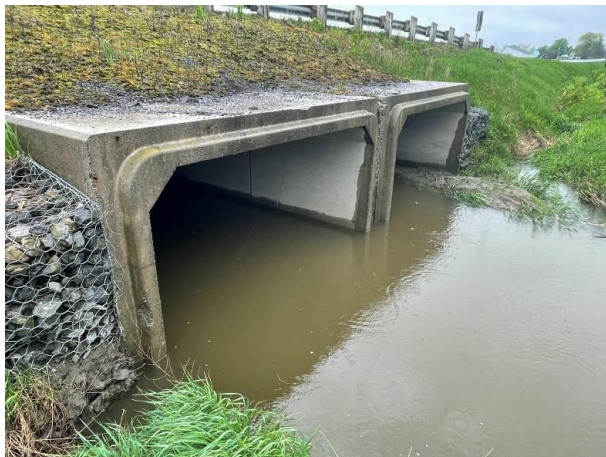
Culvert #4: Twin box culverts conveying the MacKenzie Municipal Drain. Not proposed for replacement.
