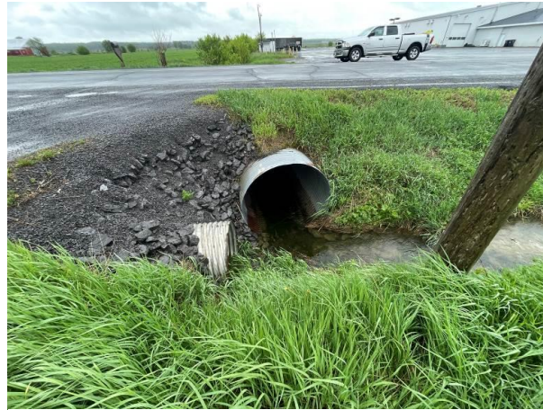
Culvert #2: Corroded, 1500 mm CSP west of 17515 CR 22. Proposed to be replaced.
