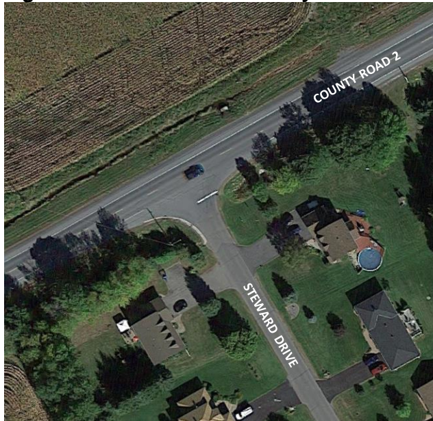
Figure 2: Aerial Photo of County Road 2/Steward Drive Intersection
